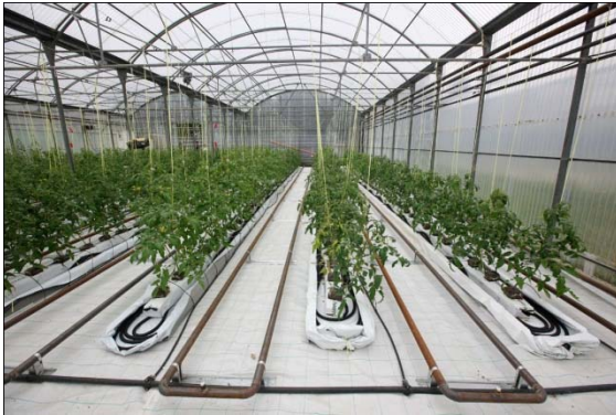
Picture 5.1 The heating system with smooth tubes [2]
