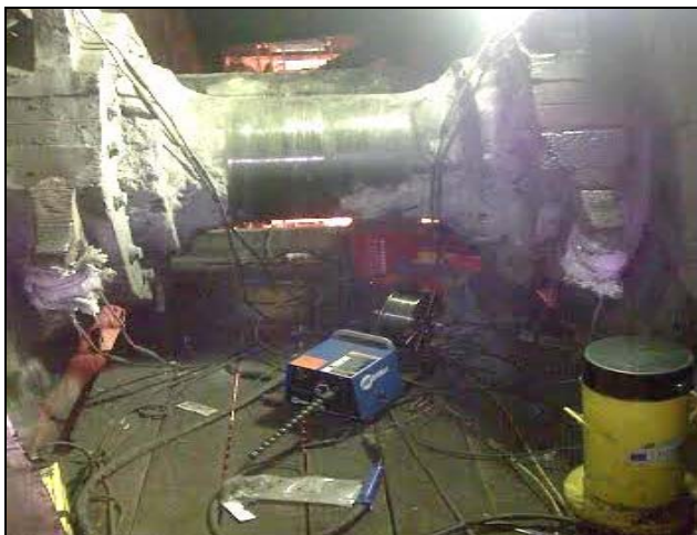
Figure 6. Electro-resistant preheating of driving wheel
